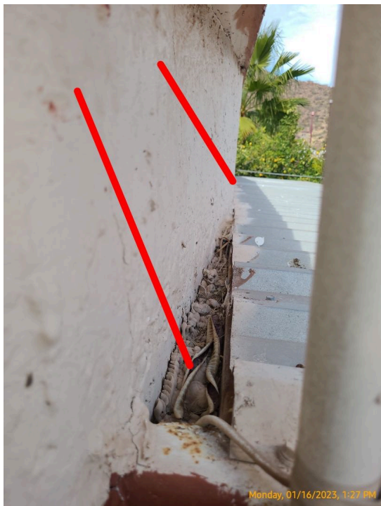
back porch no flashing/shorted
