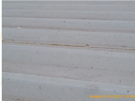
paint appears unblistered w/minimal rust
