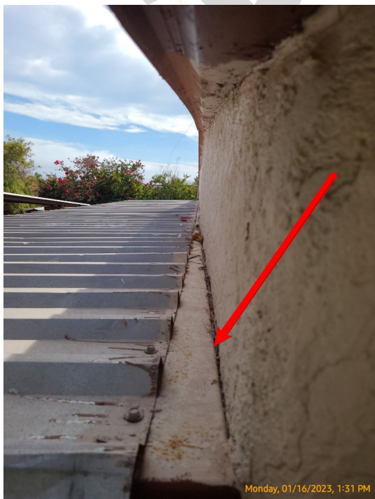
back porch north end no flashing/shorted/top view
