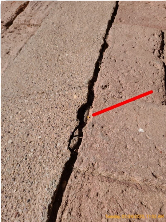
gas line visible in crack
