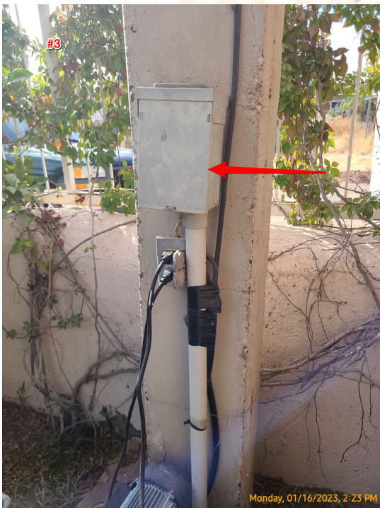
Service drop pole breaker location
