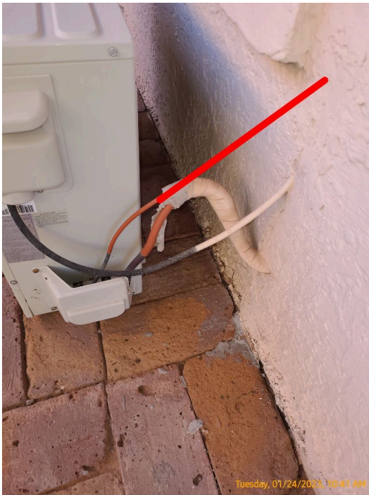
front bdrm missing insulation
