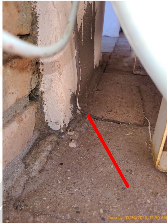
buried line. unprotected from corrosion
