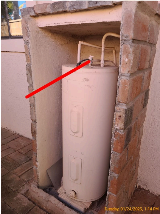
exposed no drain tube for valve
