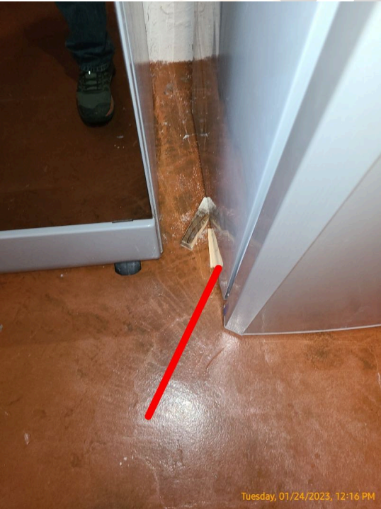
adjusting leg missing/inoperable
