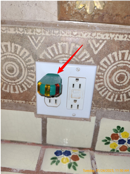
No power to this top left outlet:GFCI is functional
