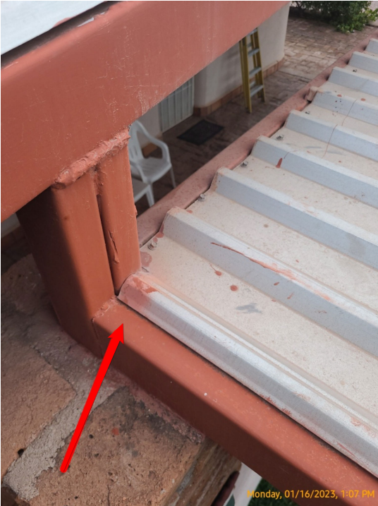
front porch north edge does not cover metal frame
