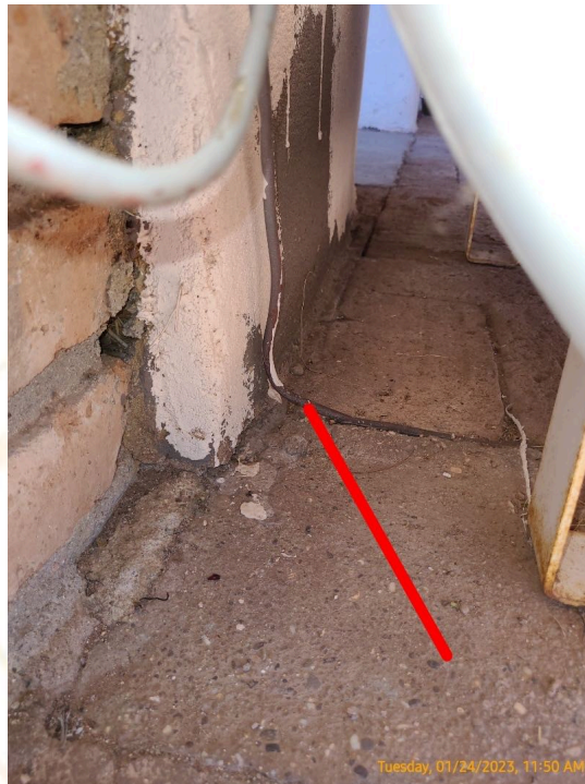
Unprotected gas line entering walkway below tank
