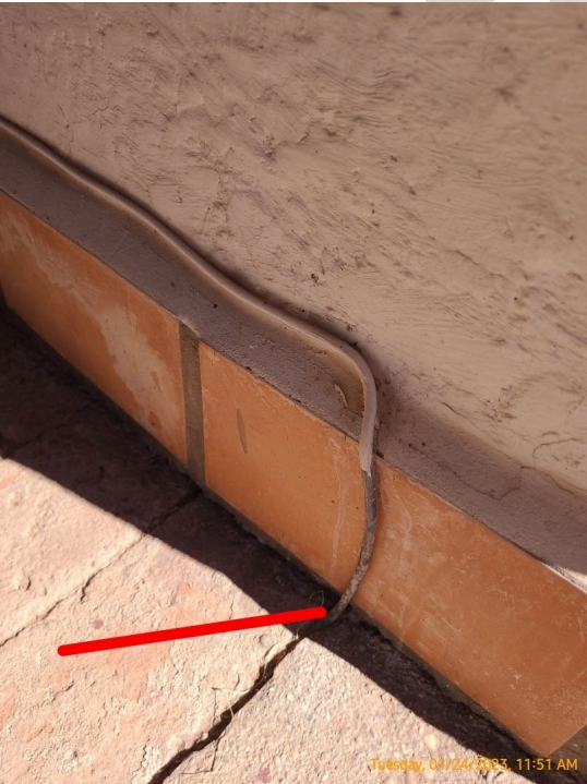
Exposed gas line adjacent to front door
